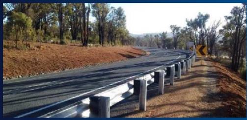
Existing two-lane road has narrow seal width, narrow gravel shoulders and steep batters
