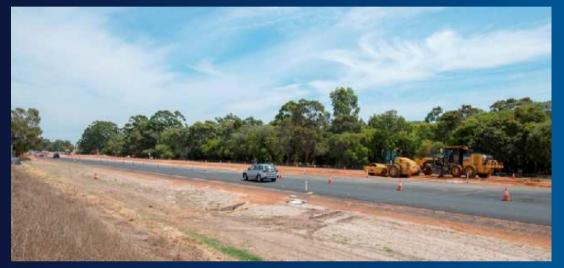
A 17km section between Capel and north of Busselton is a two lane single carriageway with passing lanes at approximately 5km intervals in each direction
